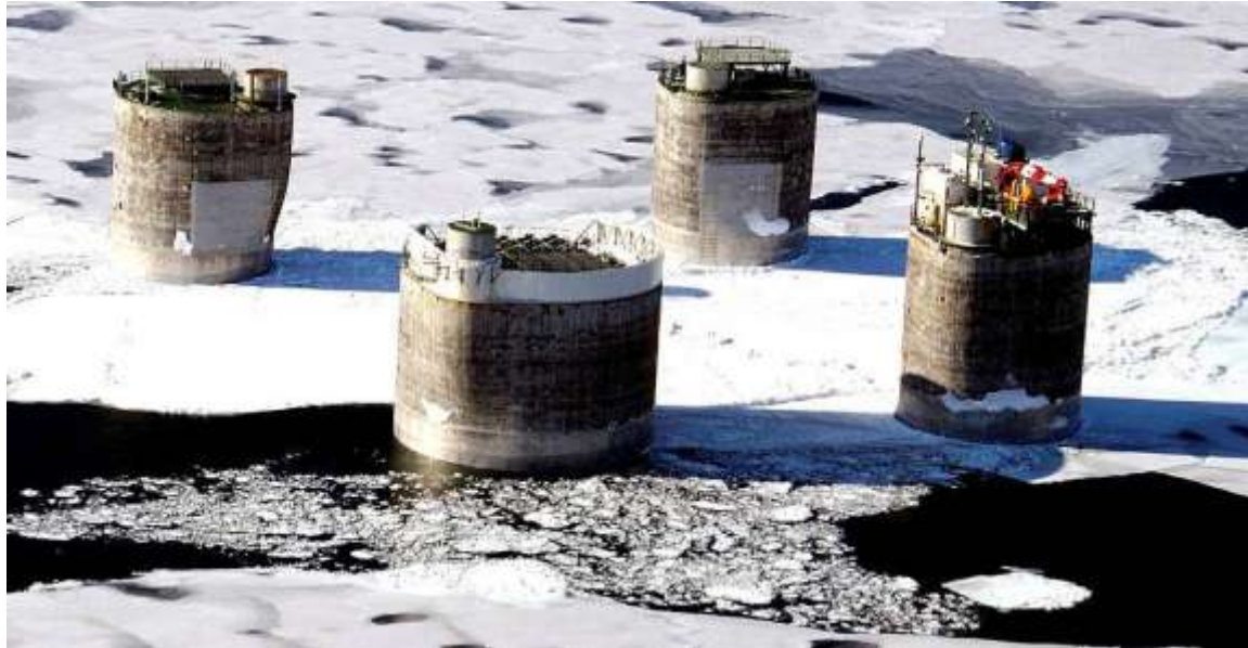
Lun-A Platform at offshore location (Sakhalin-2 Project) Photo: SEIC (Sakhalin Energy Investment Company)
